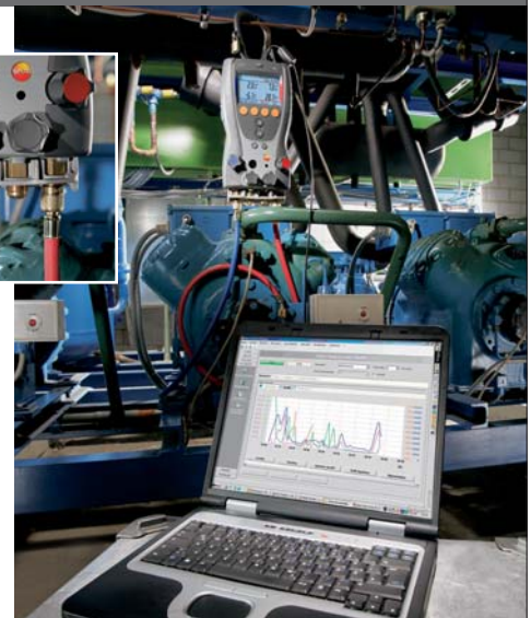
Service and maintenance on a refrigeration system using testo 556 and 560, commissioning included
