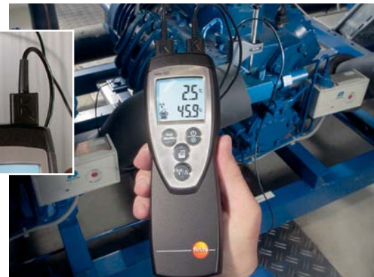
Monitoring differential temperature in compressors with pipe wrap probes
