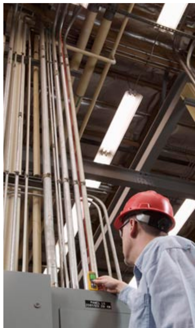
Measuring height to tall ceiling.
