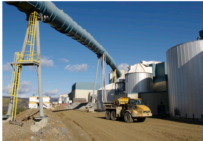
Looking north at the Mill and Filter building facilities. In the blue tube is the conveyor belt that brings the ore from underground to the mill.
