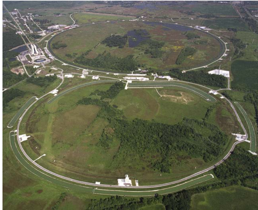
Aerial view of Fermilab Accelerators, with the Main Injector under construction in back and Tevatron in the foreground
