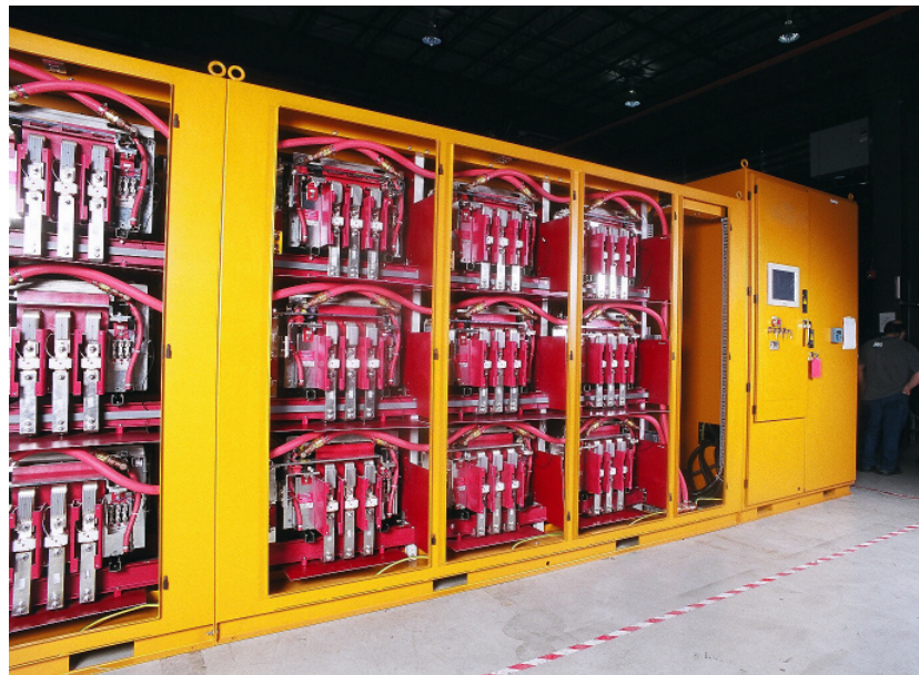
ASI Robicon Perfect Harmony water-cooled Variable Frequency Drive (VFD).
